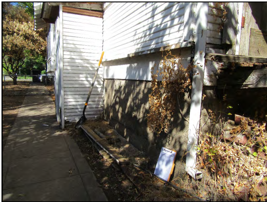
Raised concrete foundation, southern elevation (view toward west).
