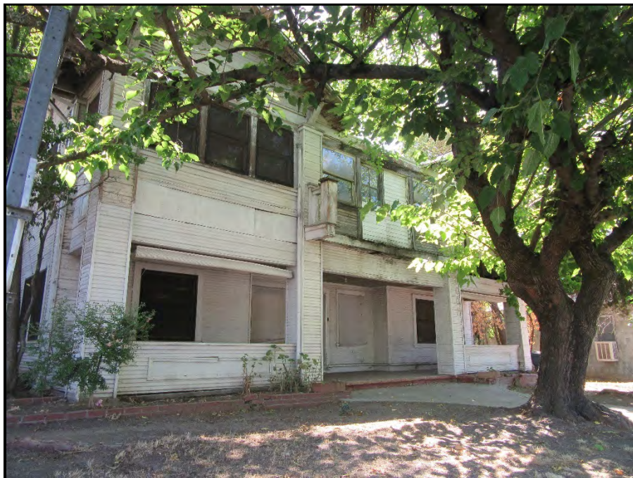
Entry of building, western elevation (view toward southeast).
