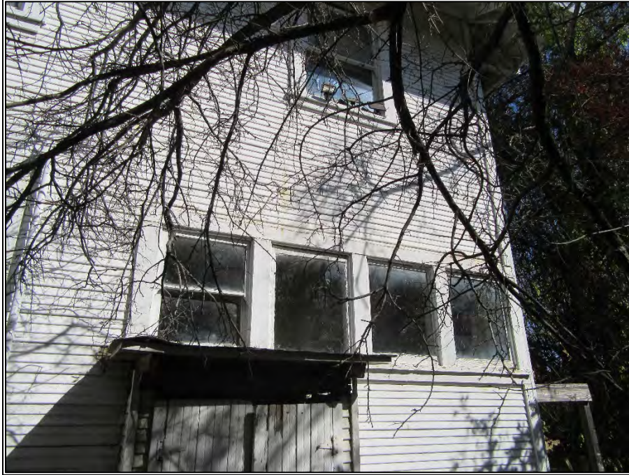
Figure 12. Wood-framed, fixed and single-hung windows, southern elevation (view toward north), September 26, 2019.
