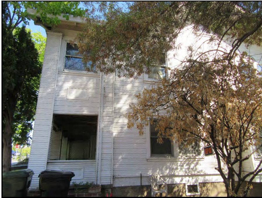
View of porch from the south, southern elevation (view toward north).
