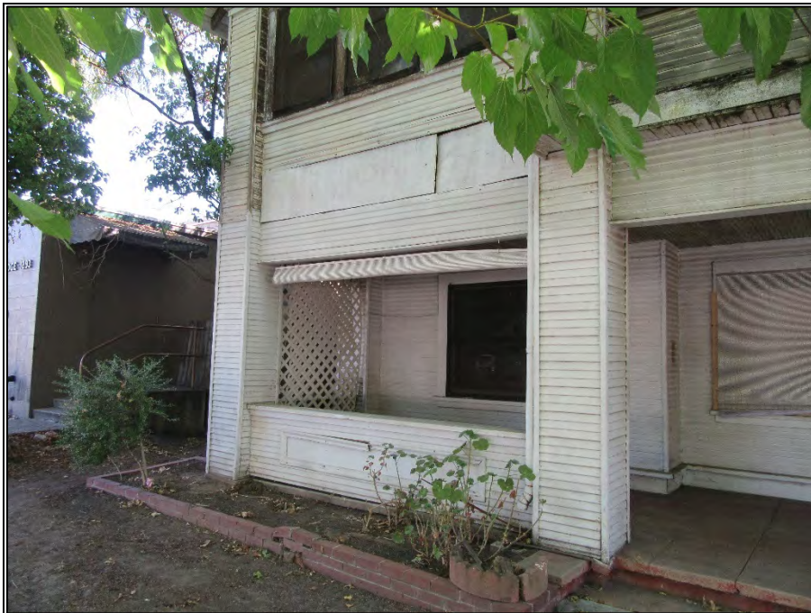
Figure 5. Front porch of building, western elevation (view toward northeast), September 26, 2019.
