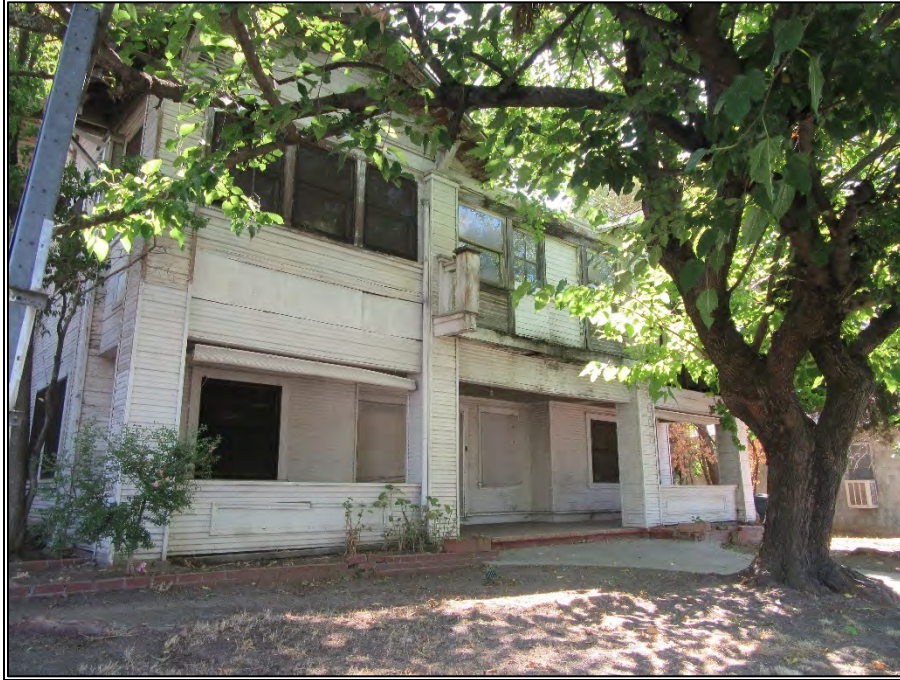
Figure 4. Entry of building, western elevation (view toward southeast), September 26, 2019.
