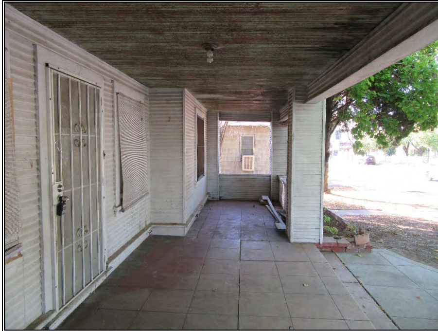
Figure 6. Front porch of building, western elevation (view toward south), September 26, 2019.
