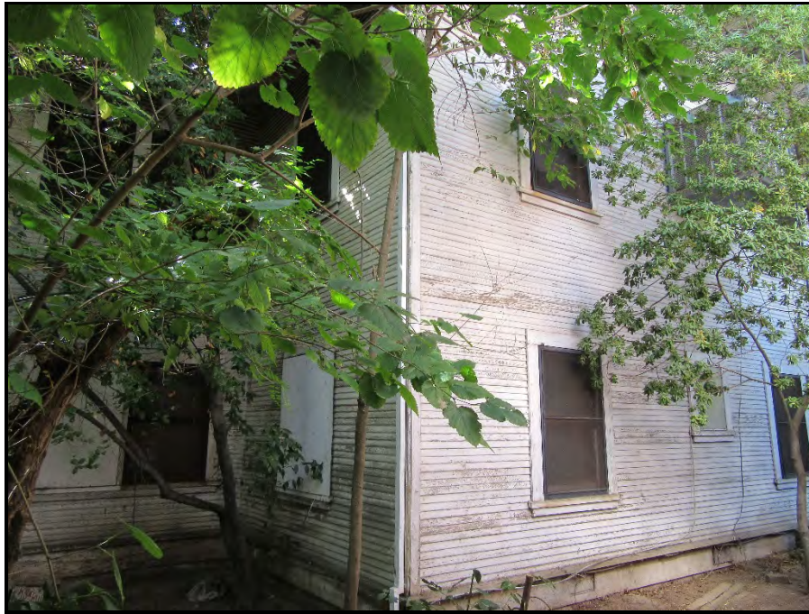
Single hung windows and horizontal siding, northern elevation (view toward southwest).
