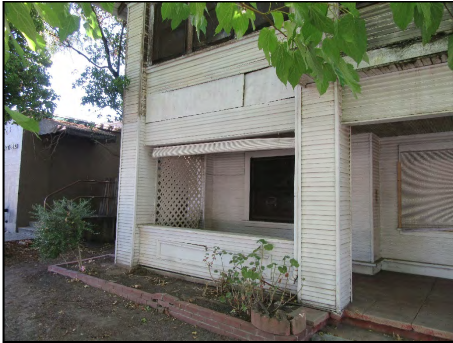
Front porch at building, western elevation (view toward northeast).
