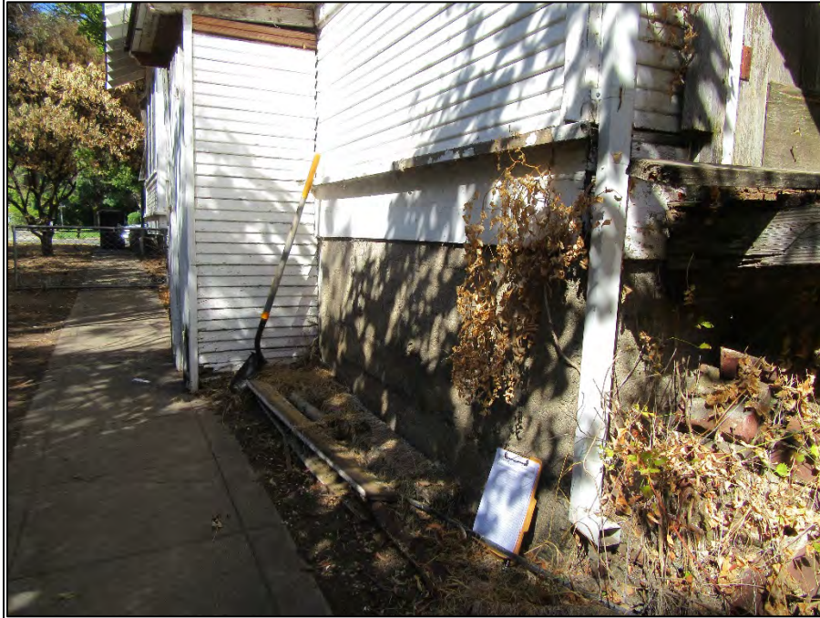
Figure 10. Raised concrete foundation, southern elevation (view toward west), September 26, 2019.
