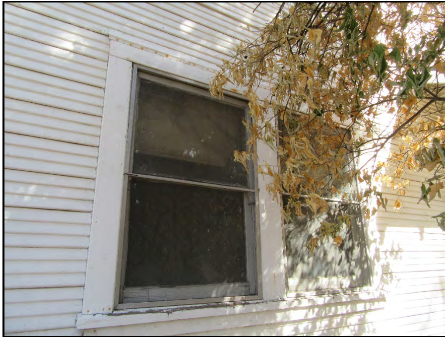
Wood framed, single hung windows, southern elevation (view toward north).
