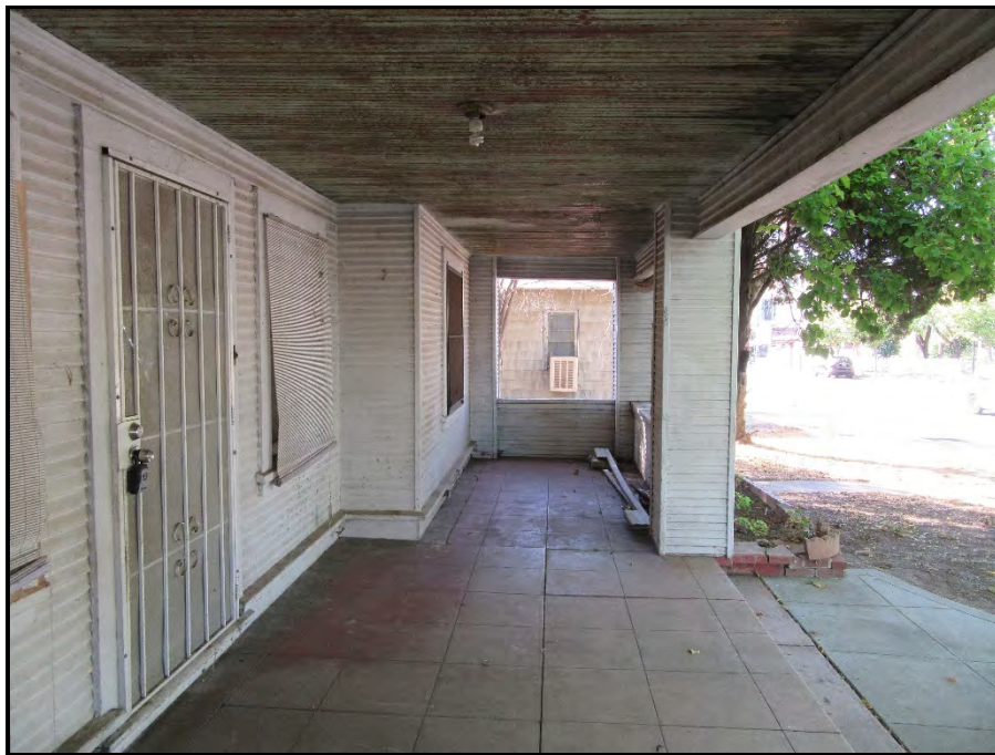
Front porch at building, western elevation (view toward south).
