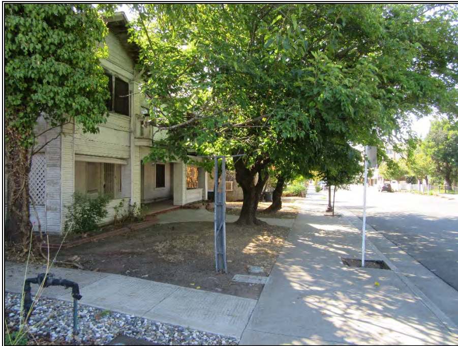
Figure 3. Front of building overview, western elevation (view toward south), September 26, 2019.
