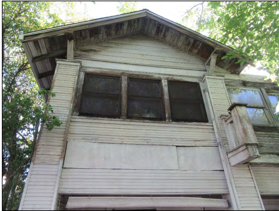
Second story windows, western elevation (view toward east).
