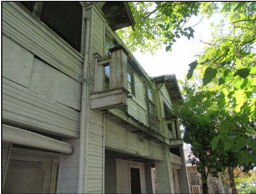
Second story, western elevation, balcony removed (view toward southeast).
