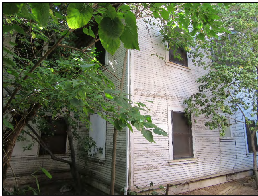
Figure 15. Single-hung windows and horizontal siding, northern elevation (view toward southwest), September 26, 2019.
