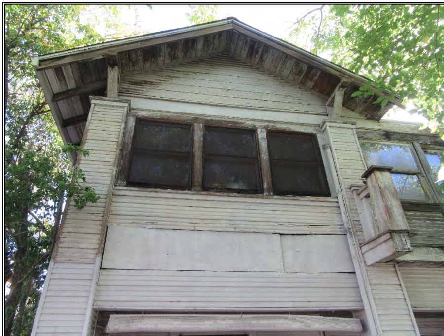
Figure 7. Second-story windows, western elevation (view toward east), September 26, 2019.
