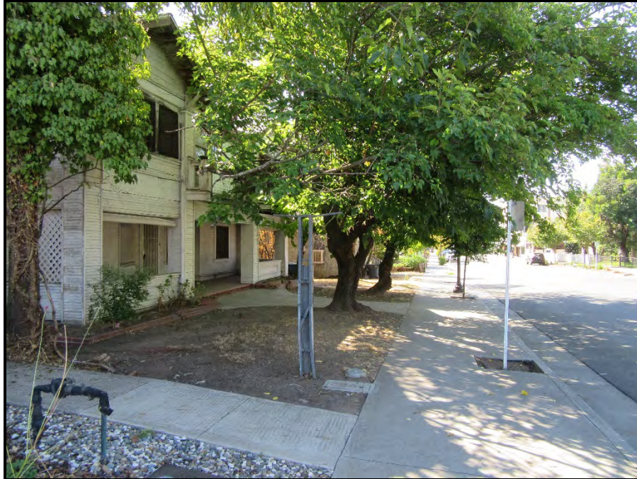
Front of building overview, eastern elevation (view toward south).
