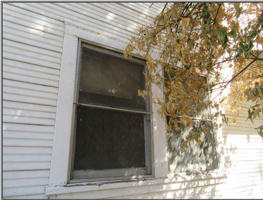
Figure 13. Wood-framed, single-hung windows, southern elevation (view toward north), September 26, 2019.
