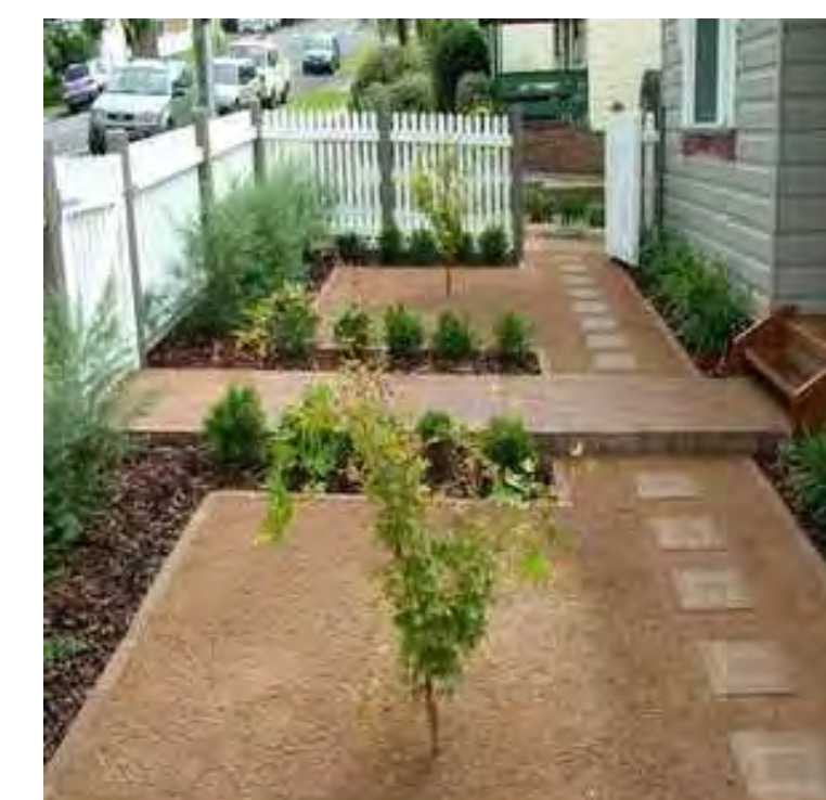
6' Stabilized decomposed granite paving
