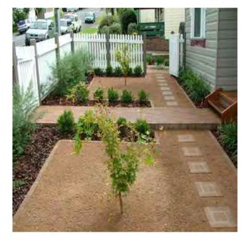
6' Stabilized decomposed granite paving
