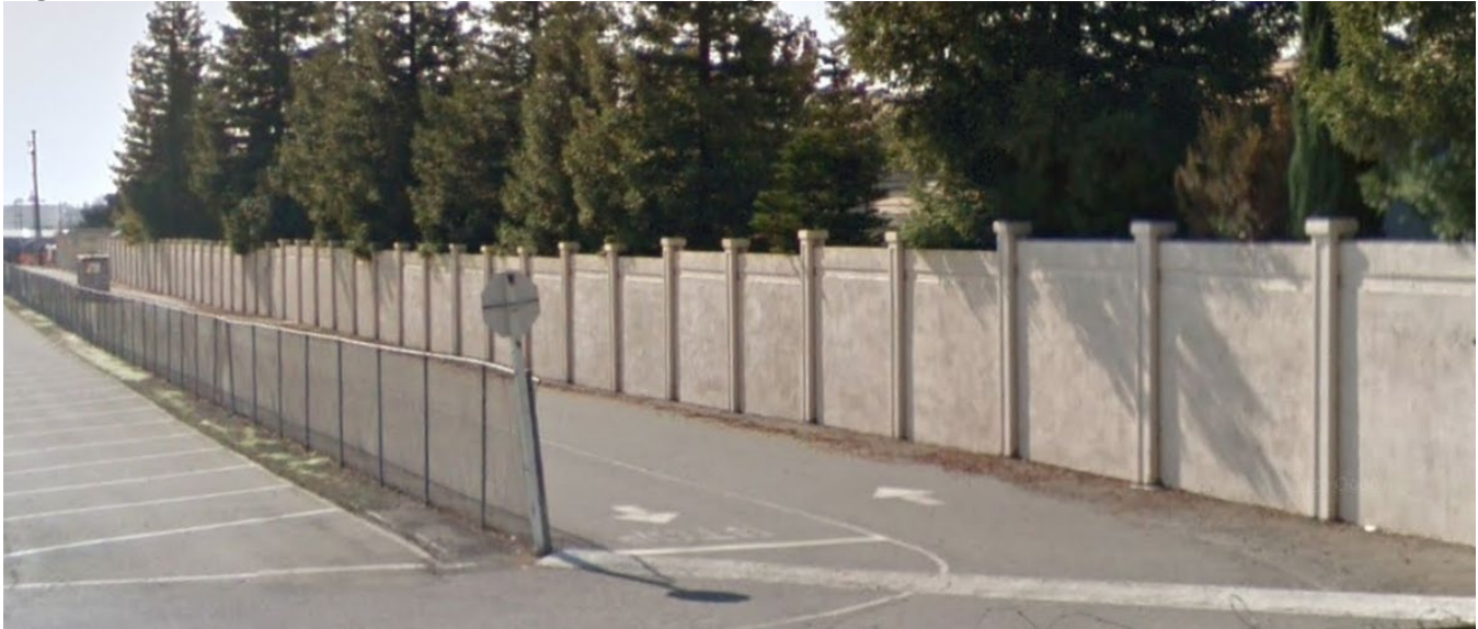
Figure 3. View from North into the Site of Existing Screen Wall on West Property Line
