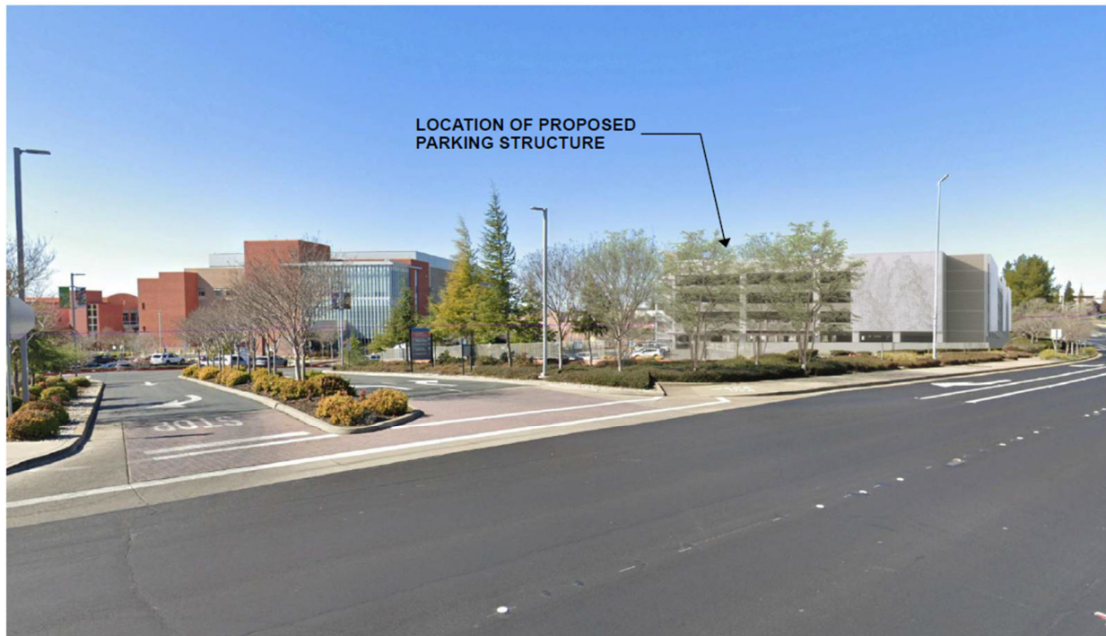
Figure 5: View from northbound Eureka Rd.
