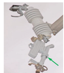
S&C Fault Tamer Fuse - Open
