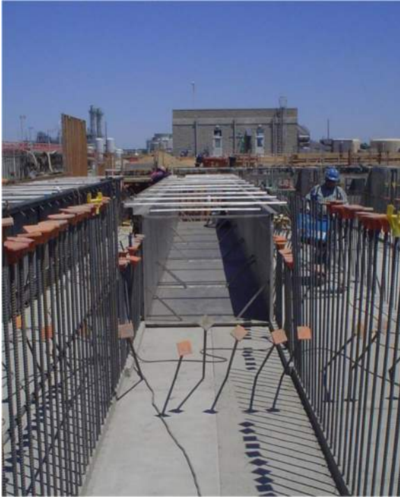
Previously installed channel liners at Pleasant Grove WWTP UV channels.
