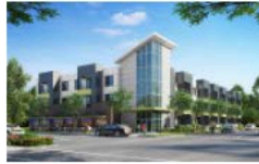
3rd & S Apartments, Sacramento CA
