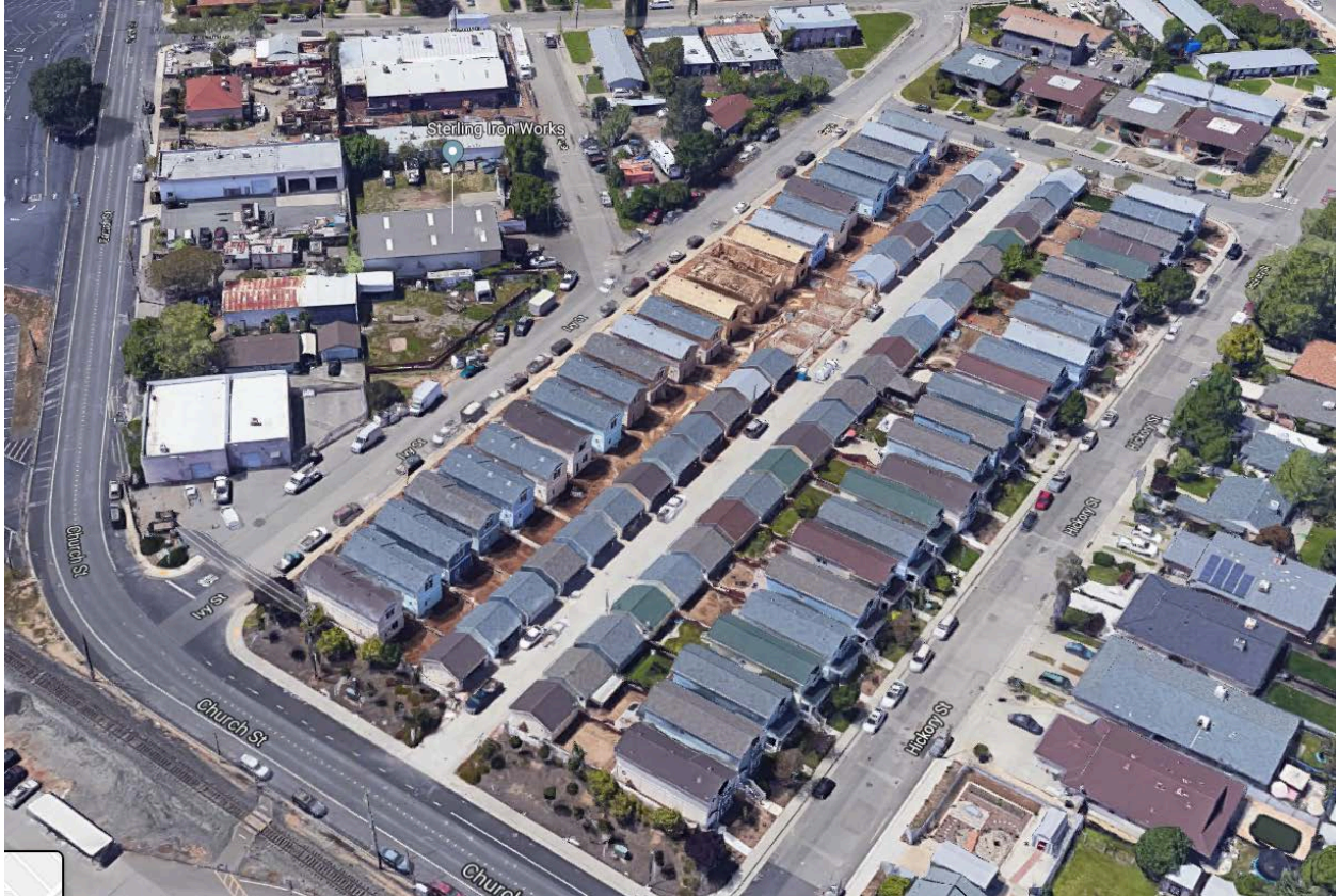
Hickory and Church Row Houses
