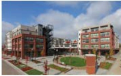
Cannery Place, Sacramento CA: Apartments and Commercial
