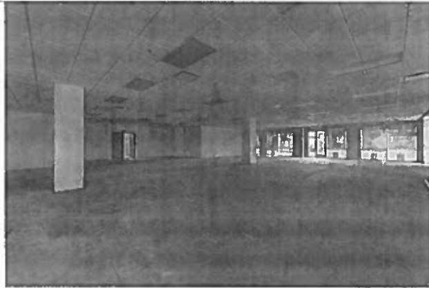
TYPICAL UNIT INTERIOR
