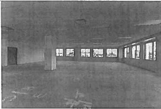
TYPICAL UNIT INTERIOR
