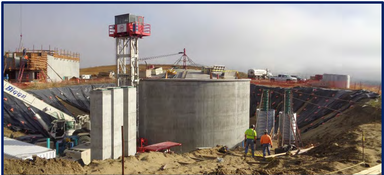
Figure 1: View of a pre-stressed concrete water storage tank, with encased pump cans in the foreground, under construction at the West Hills Water Treatment Plant in Hollister, CA. Auburn Constructors was the prime contractor on this $27.8M contract.
