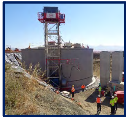
Figure 5: View of one of DN Tanks' pre-stressing machines wrapping a concrete tank.
