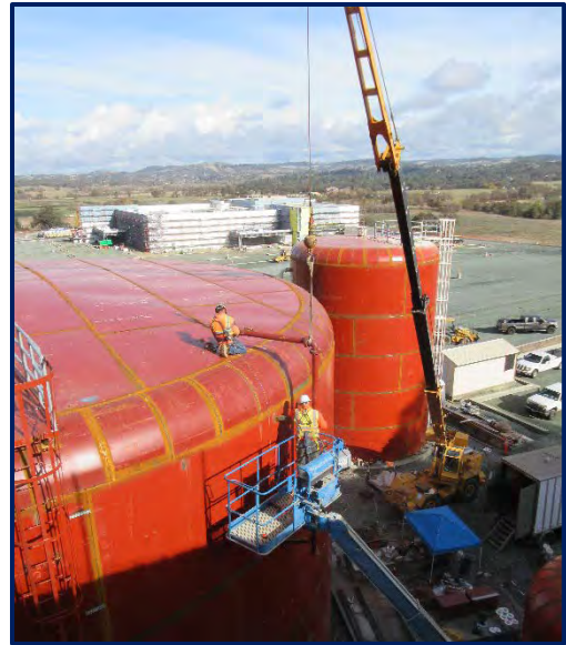
Figure 14: Auburn crews installing tank piping on a steel PW storage tank for Harrah's NorCal casino.
