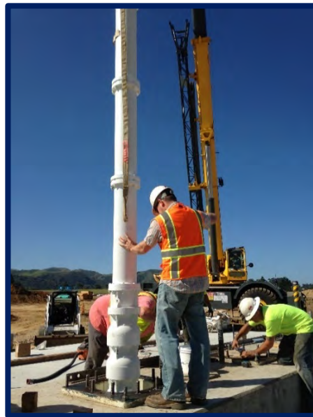
Figure 11: Auburn personnel installing vertical turbine pumps at the Los Osos Water Recycling Facility Project.
