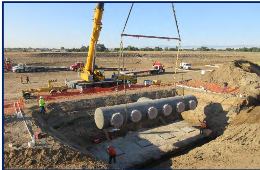
Figure 15: Auburn crew installs a 72" cement coated steel pipe manifold in Lathrop, CA.
