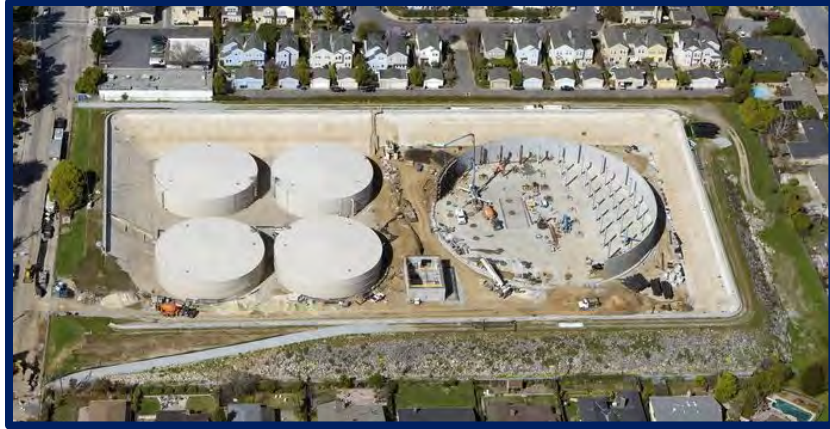
Figure 13: Aerial view of the Bay Street Reservoir Replacement - Phase 2 project in Santa Cruz, CA constructed by Gateway Pacific. This project included the construction of a 6MG prestressed concrete potable water storage tank.
