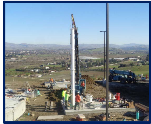
Figure 16: Auburn crew installing vertical turbine pumps at the West Hills Water Treatment Plant.
